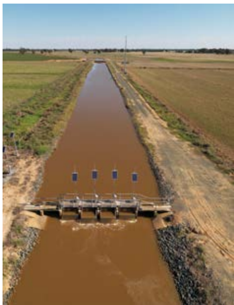
Channel modernisation through automation has contributed significantly to improving system efficiency and cutting losses resulting from water flowing out of the system unused.
